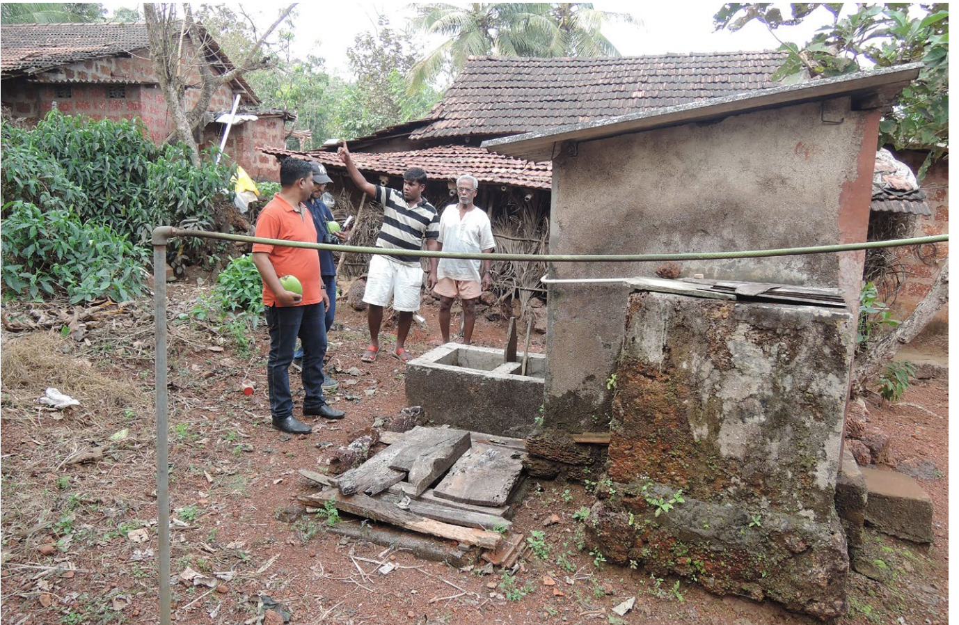
Top; A ‘modern’ house built by a family residing in Mumbai on their ancestral land in Kondhe. Bottom; Bandhu shows a system promoted a couple of decades back by the government to produce biogas for cooking with cow dung.
