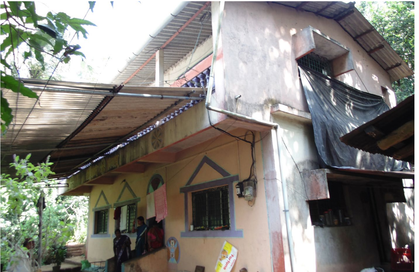
Top; The Mohite family home has two kitchens. The modern one is inside the house, the other traditional one is inside the structure pictured. Bottom; The Kule house in Kondhe is a two storey brick and concrete structure.
