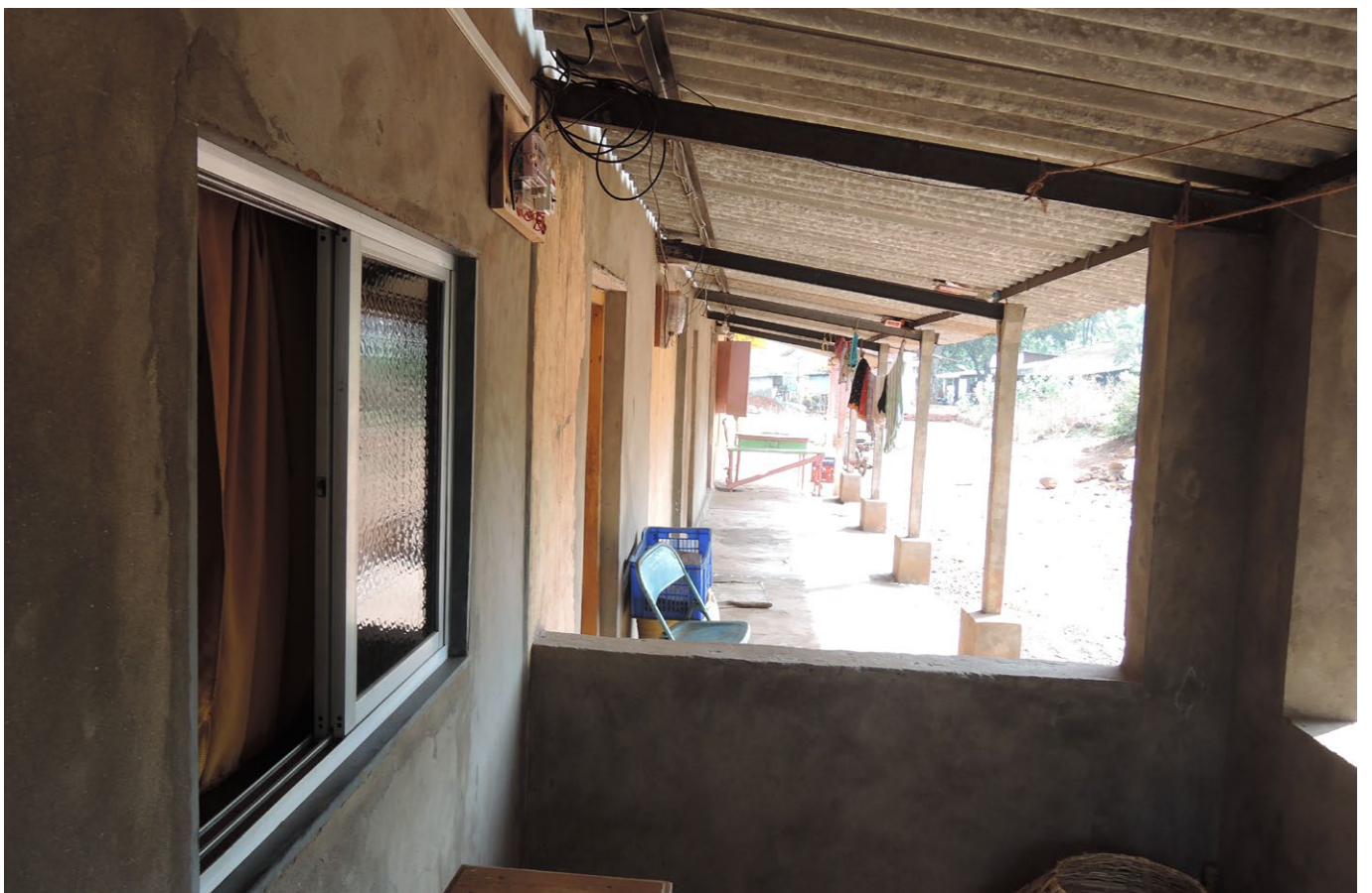
Top ; A chawl-like structure in Kondhe with rooms for rent that can be used either as shops or residences. Bhandu Mohite is the owner of the structure that he developed on his family's land. He prefers to live in one of the rooms in the structure rather than his ancestral home, which is much bigger. Bottom ; A close up view of the front of the chawl-like structure.
